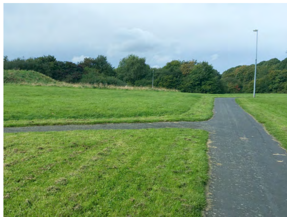
10. Lack of directional signage - existing footpath cycleway towards Halton Lea.
