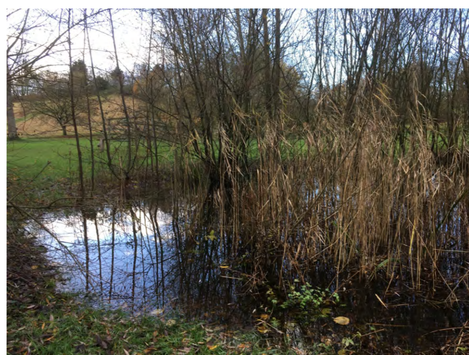
18. Overgrown vegetation obscuring and reducing capacity of ponds.
