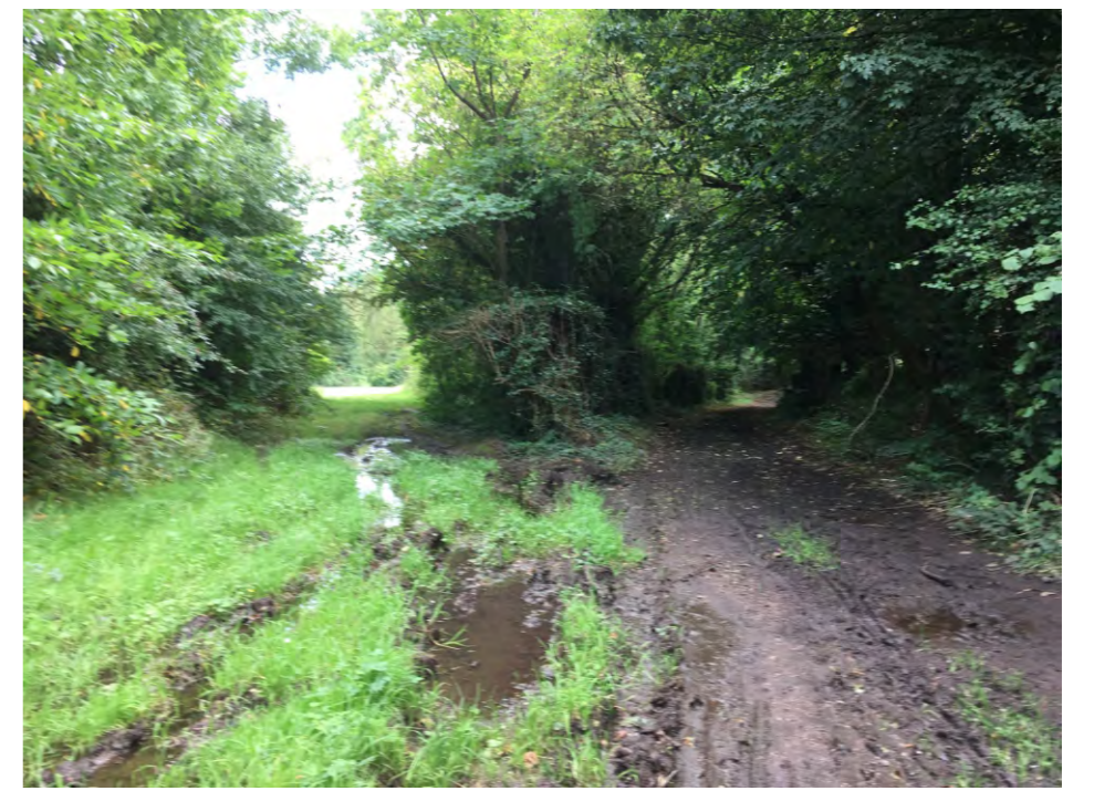
4. Lack of path surfacing connecting routes through the park.
