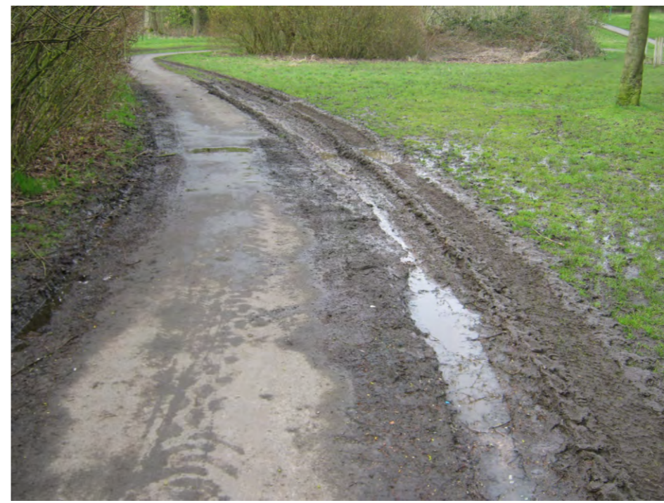
3. Existing path surfacing of insufficient width to allow for maintenance access through the park.
